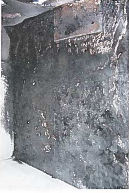
FIGURE 8-13 Pattern on floor showing intense charring of plywood and irregular destruction of carpet and pad, which is most extensive at the door. Photo courtesy of Special Agent Mike Marquardt, CFI, ATF, Grand Rapids, MI. Test courtesy of the Iowa Chapter of the IAAI.
